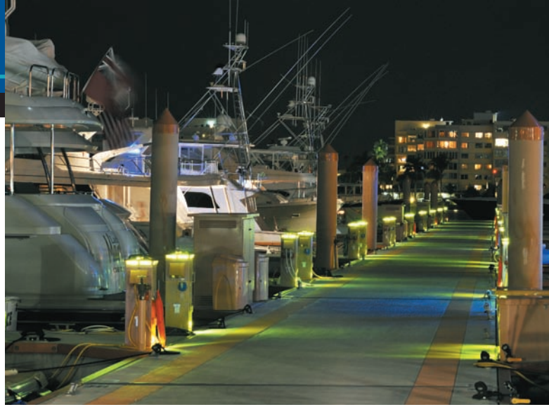
Palm Harbor Marina keeps its new concrete docks well lit at night to prevent tripping hazards.
